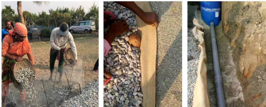
Figure 5: Construction of gabions (left), jute lining and filter gravel (middle), abstraction drain (right)
