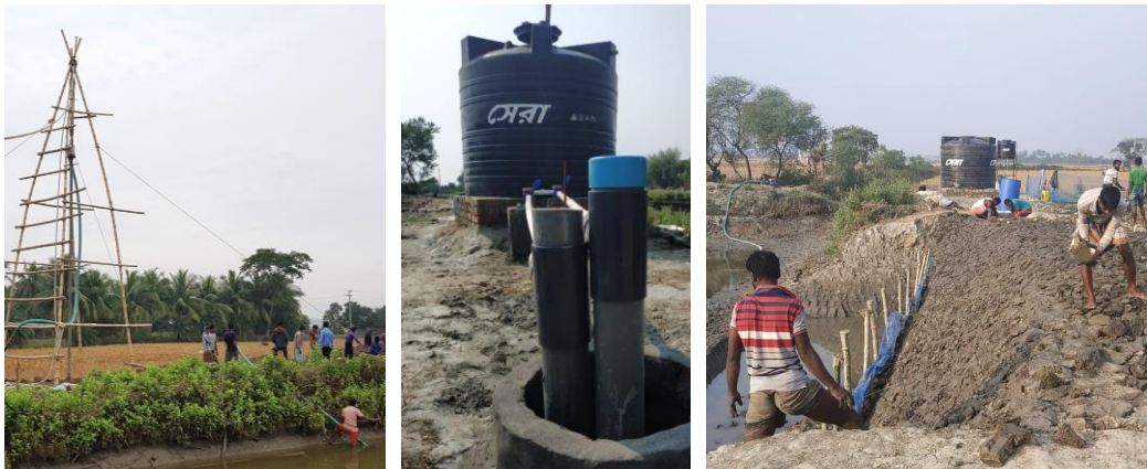
Figure 3: Drilling of the MAR well (left), installed well and infiltration reservoir (middle), construction of drain intake (right)
